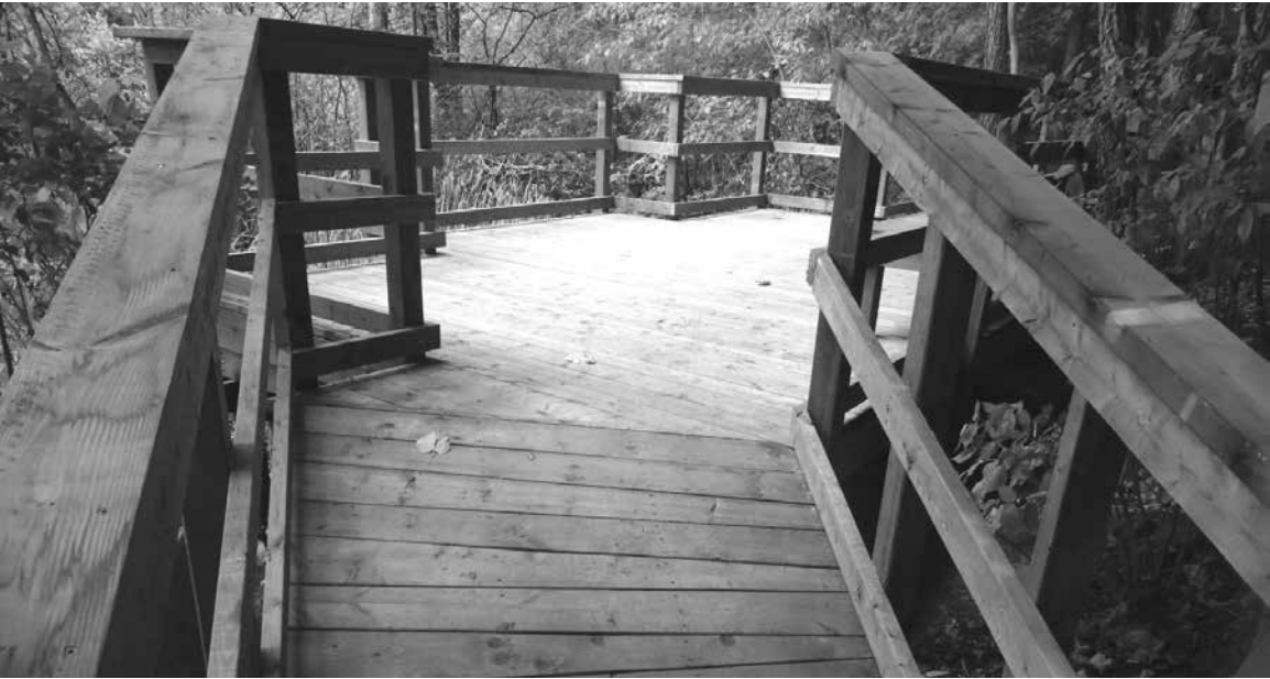
For the second time in a year, the city has replaced a decaying bridge along the Caldwell-Carver Conservation Area trail with an expanded version, allowing for a better viewing area.
