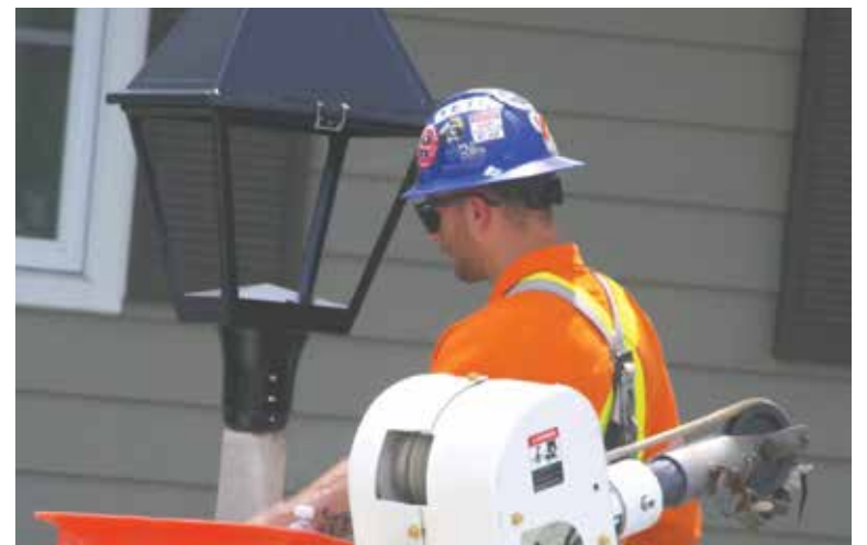
IN WITH THE NEW ... A new LED light fixture is installed on that same pole. A total of 144 street lights, some possibly dating back 70 years, were updated this summer.
