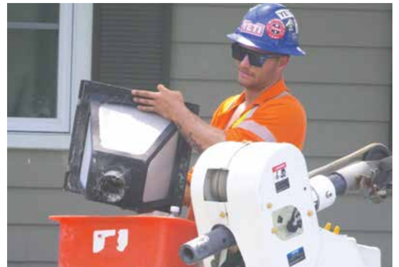
OUT WITH THE OLD ... A city employee removes one of Manor Park's old street light fixtures in front of a home on Dunloe Avenue. PHOTOS: EVAN BROWNE
