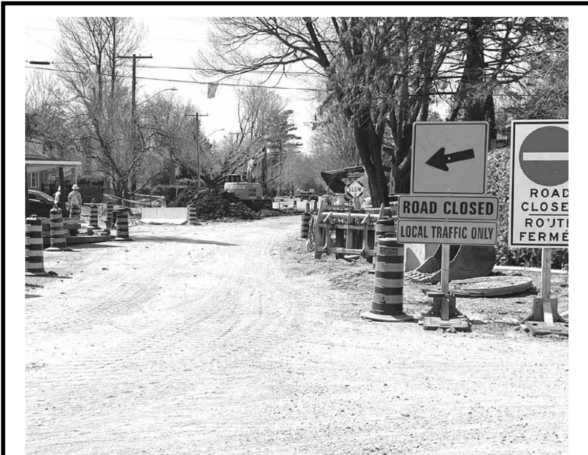
This promises to be a busy construction season in and around Manor Park. In addition to the ongoing integrated renewal project on six streets (Finter, Arundel, Kilbarry, Jeffrey, Farnham and Braemar), Enbridge will be working to replace gas pipelines along Sandridge and St. Laurent Blvd. over the next several months. This photo shows road work at the intersection of Kilbarry Crescent and Arundel Avenue.
