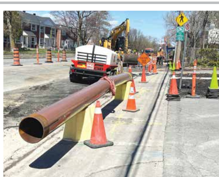
Enbridge Gas has already begun to replace the gas line along St. Laurent Boulevard. Here, this work was taking place between Quelque Chose Patisserie and Bread and Roses Bakery on May 1. PHOTO: RYLAND COYNE
