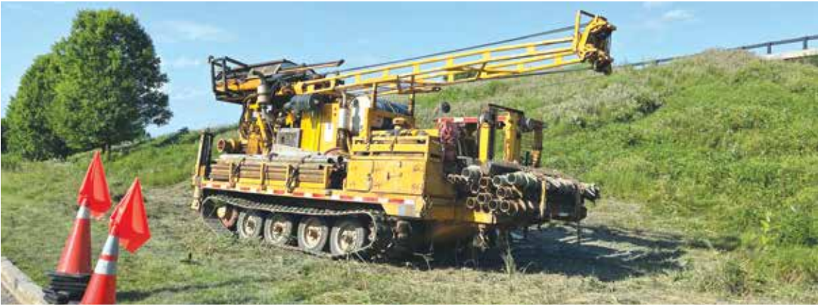
Workers have drilled bore holes at various sites along the Aviation Parkway to determine the feasibility of widening the road to four lanes. PHOTO: SUBMITTED
